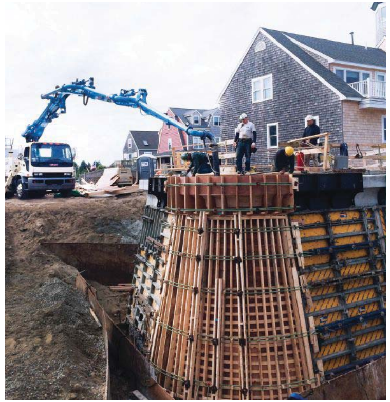
The 20Z-meter handles intricate concrete placement.
