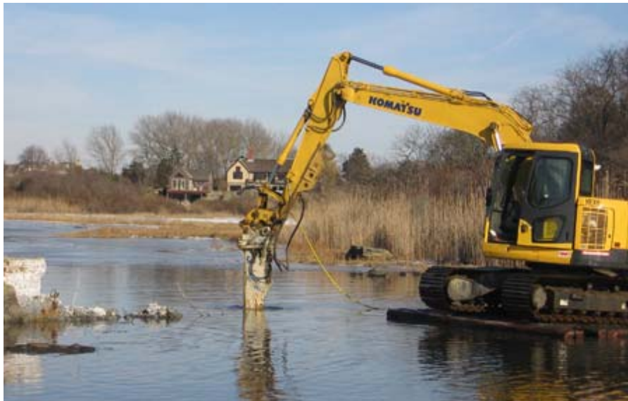
January 26, 2009: Northern Construction Service removes the central dam from Gooseneck Cove.
