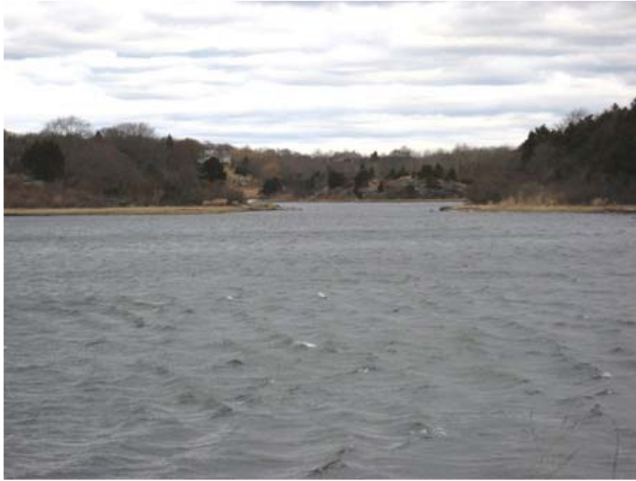
February 12, 2009: The dam at Gooseneck Cove is completely gone!
