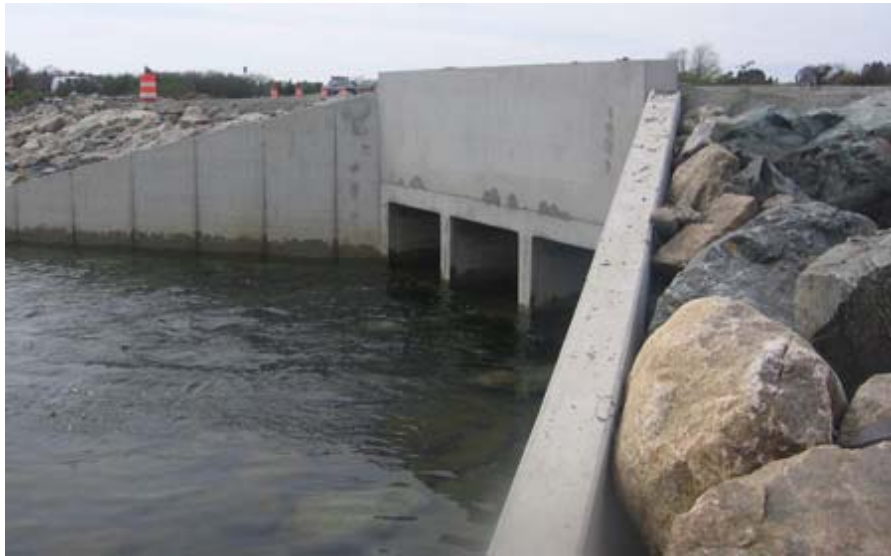
April 6, 2009: The Ocean Drive culvert has been installed beneath Hazard Road.
