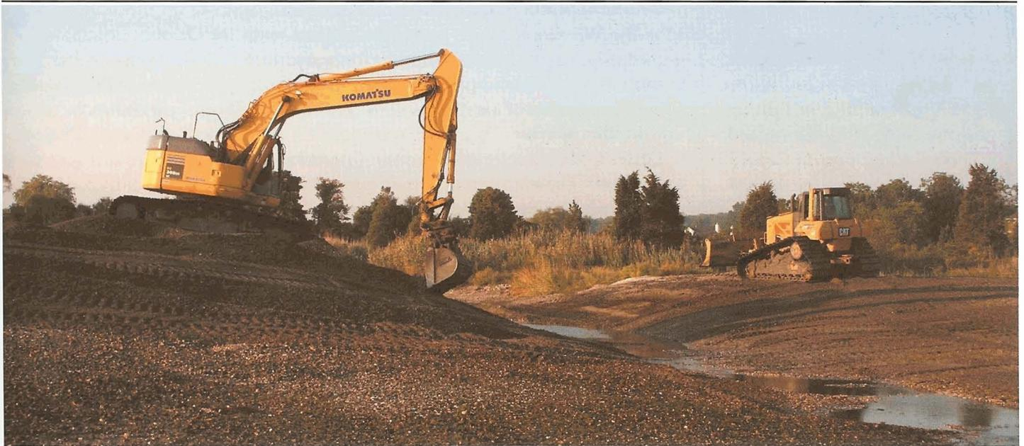
*Contractors remove the dirt plug so that tidal water can flood Town Pond in Rhode Island.*
